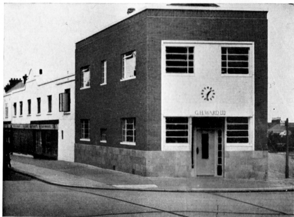
Our Canterbury Street Offices
